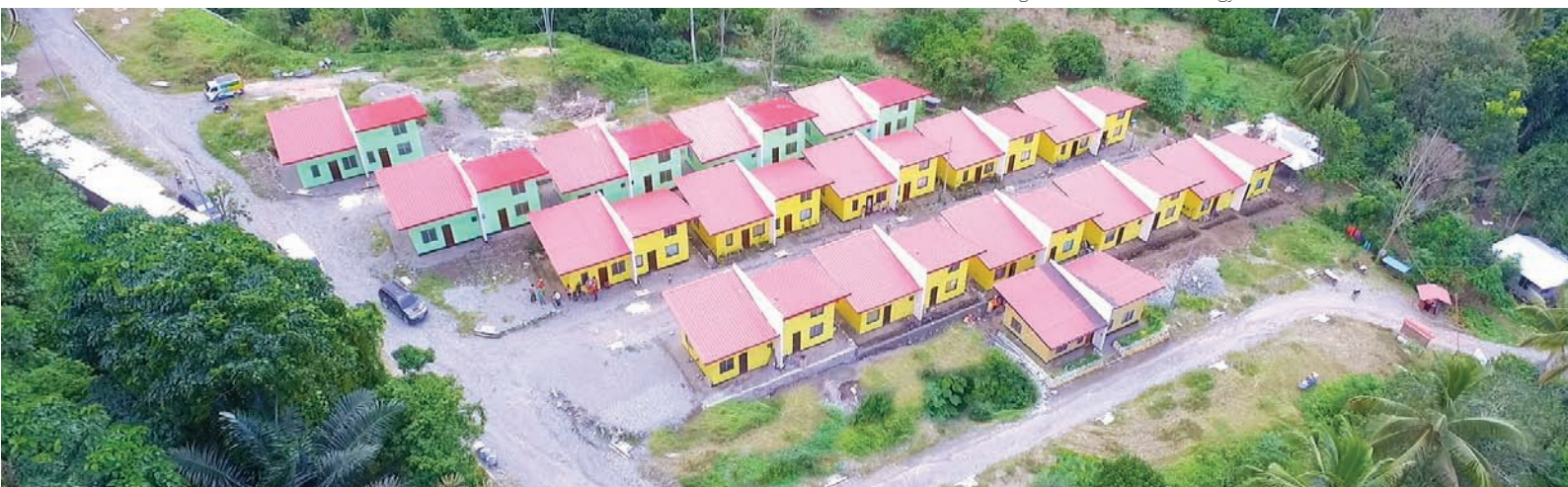
Housing units constructed at Brgy. Elizalde relocation site
