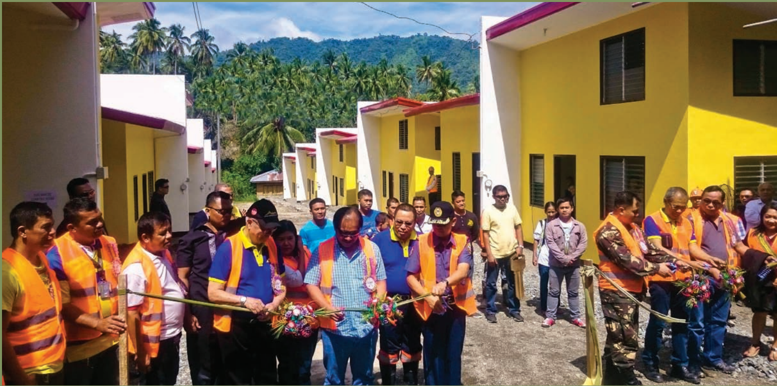
Turnover of first 20 housing units in Brgy. Elizalde
