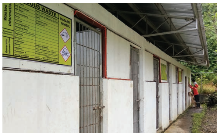
Hazardous Waste Storage Facility
