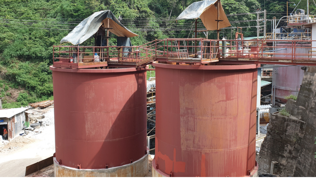
Completed 2 units 21'x22' leach tank for 200TPD.
