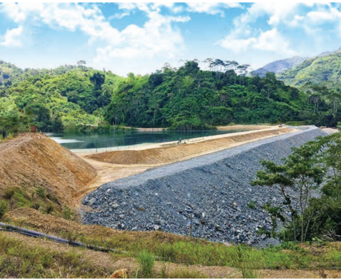
Maco Tailings Management Facility
