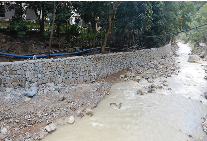
River bank protection
