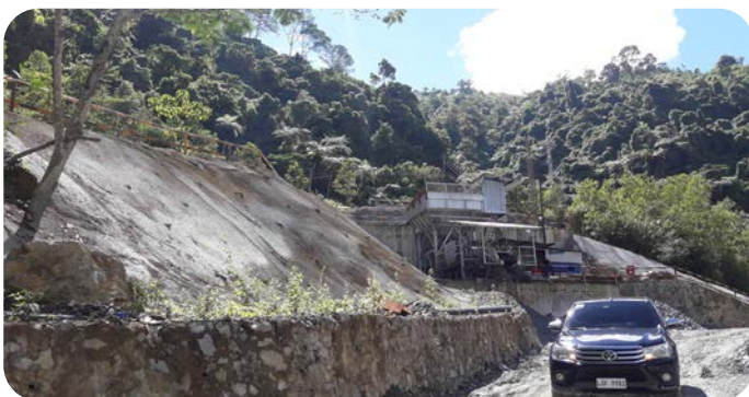
Shotcreting at Level 2 crushing area.
