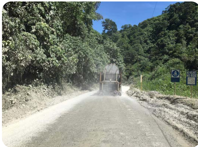
Water spraying of road surface
